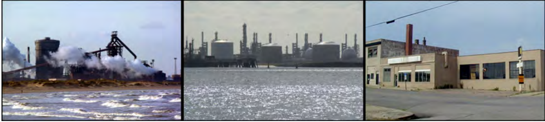
FIGURE 5.5: Industrial land use. Left: heavy industry by the seaside [Britton 2001e]. Center: heavy industry by the river [Britton 2001f]. Right: light industry [Urban Properties 2001].
